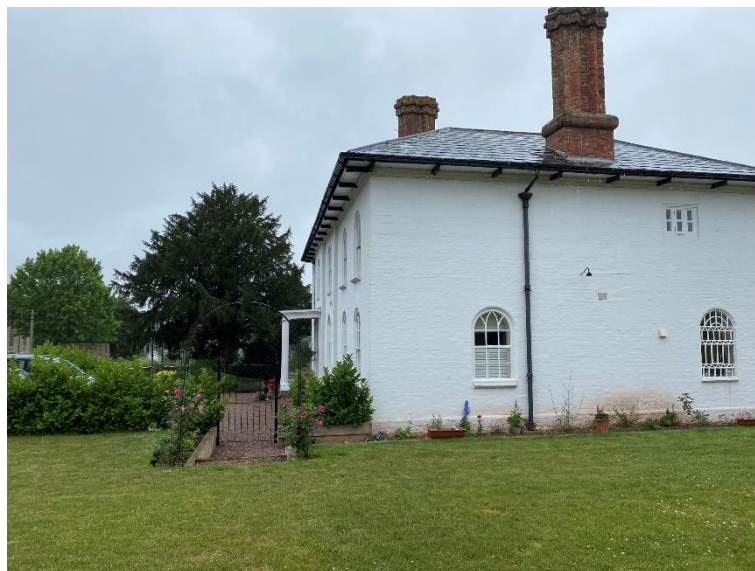
Site photo showing the side (east) elevation of Porch House, which faces the site of the dwelling.
