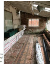
Image 5: Internal view of the Glass House showing Godwin floor tiles and deflection to the roof structure over
