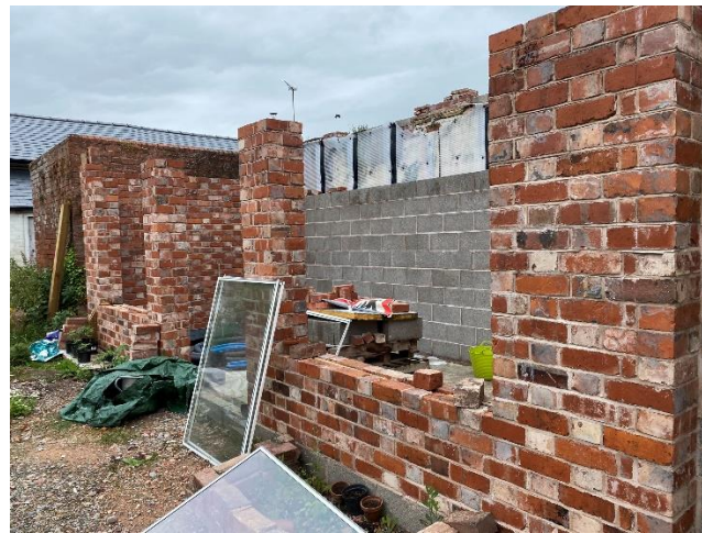
Site photo of partially reconstructed Glass House (July 2020)
