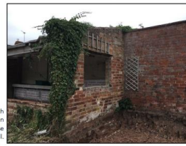
Image 7: Eastern elevation which clearly shows the difference in brickwork between the Glass House and boundary wall.
